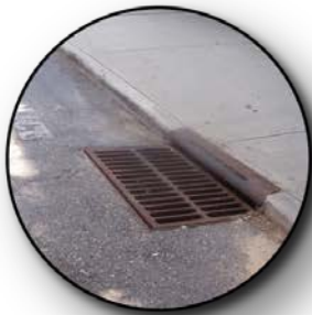
Curb and Gutter / Storm Drain (Closed System)
