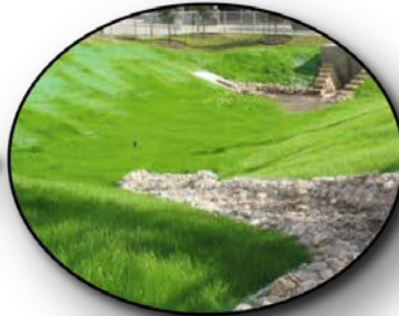
Grass Detention Area (Wet Pond planted with Fescue Grass)
