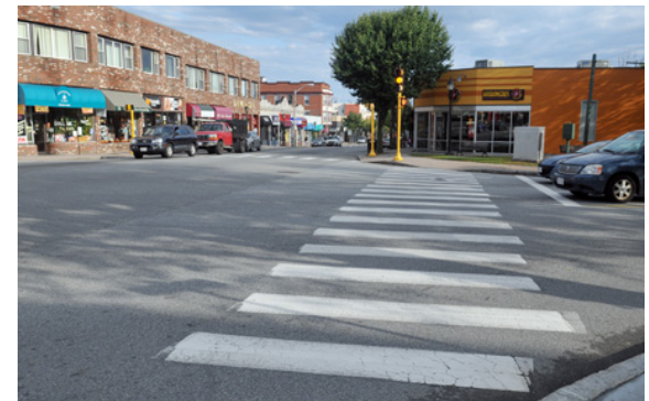
Ladder Crosswalk with Stop Line
