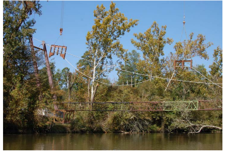
Cable Placement with Idlers
