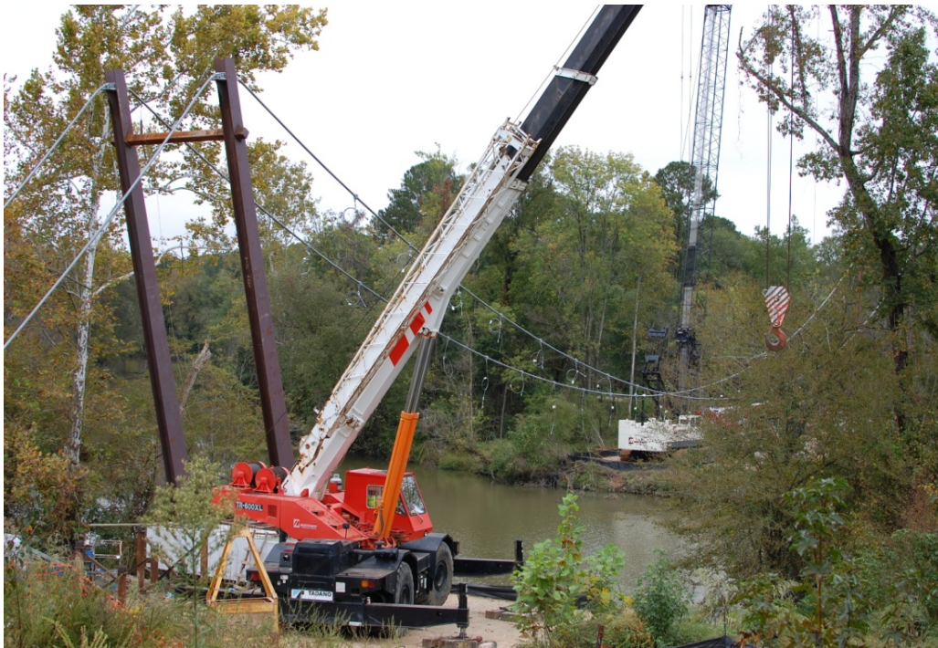
Suspender Cable Placement
