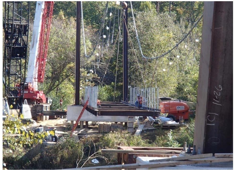
Steel framing underway
